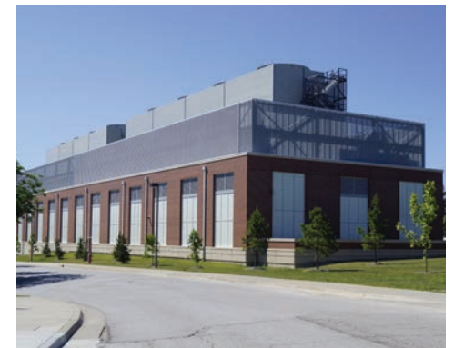
East Campus Chilled Water Plant
