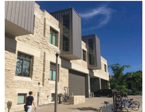
The MU Student Center masks its loading dock area behind service doors.
