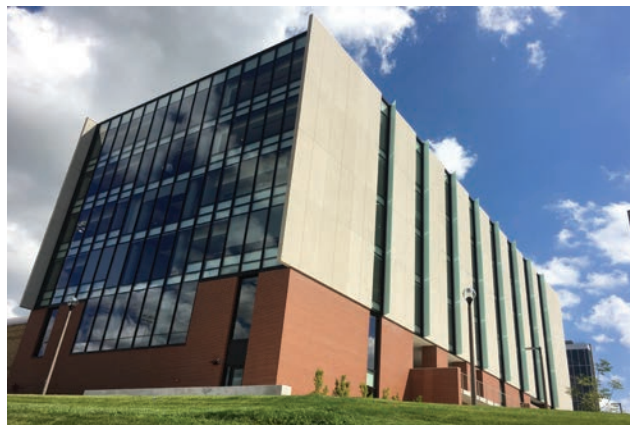
The south and west facades of PCCLC minimize solar gain and employ vertical shading fins, while glazing is maximized on the north and south facades. The south facade is additionally served by tuned horizontal louvers to harvest daylighting.
