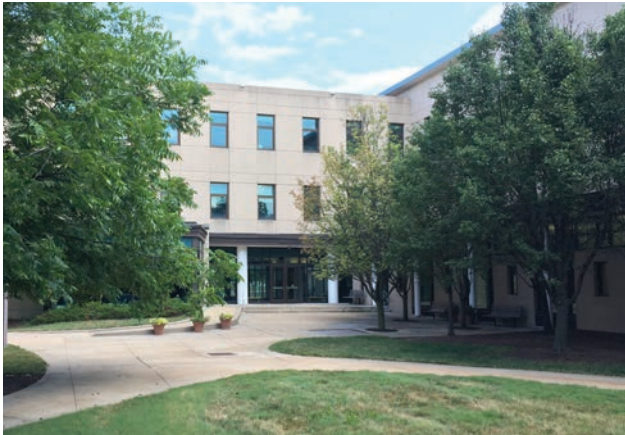
The entry vestibule to the Anheuser Busch Natural Resources building intentionally connects the indoor learning space with the outdoor Woodland Garden.
