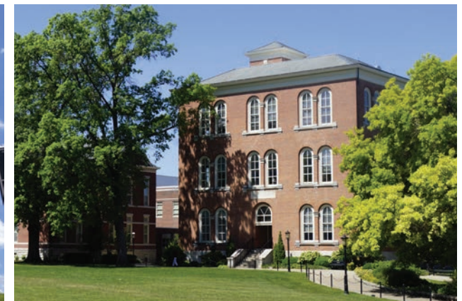
Switzler Hall's renovation and addition allowed a more efficient reuse of a historic building and also supports campus walkability and compactness.
