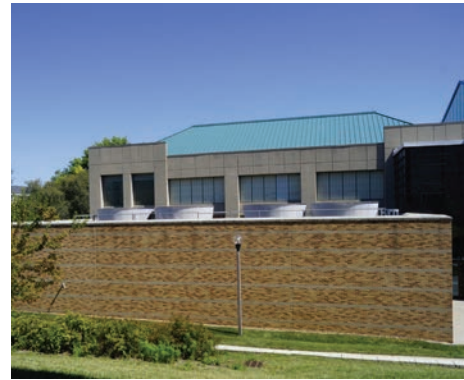
The Student Recreation Complex screens its cooling towers behind a brick landscape wall.
