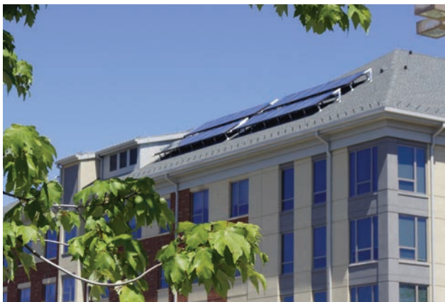
Brooks Hall solar panels for residence hall domestic water heating.
